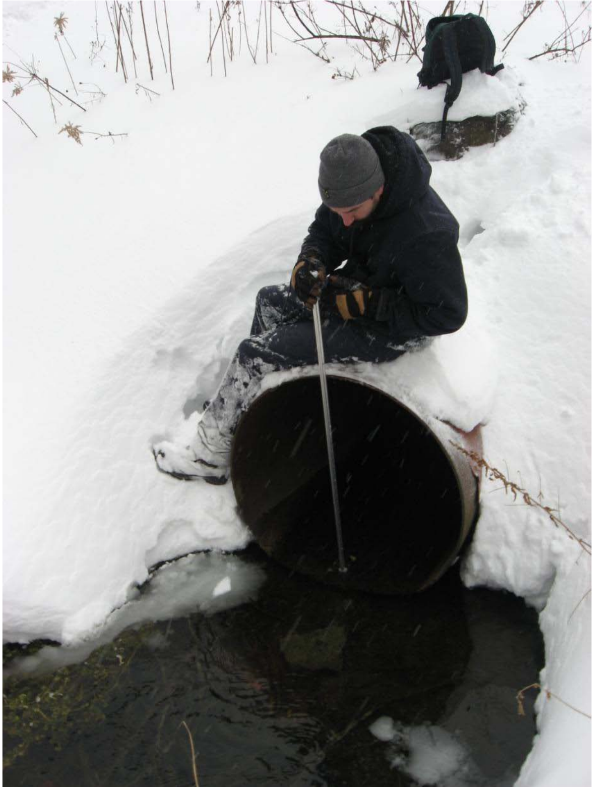
Wintertime flow measurements through a culvert for initial site assessment. Approximately 15 site assessments were done to identify the best candidates for the hydro systems.
