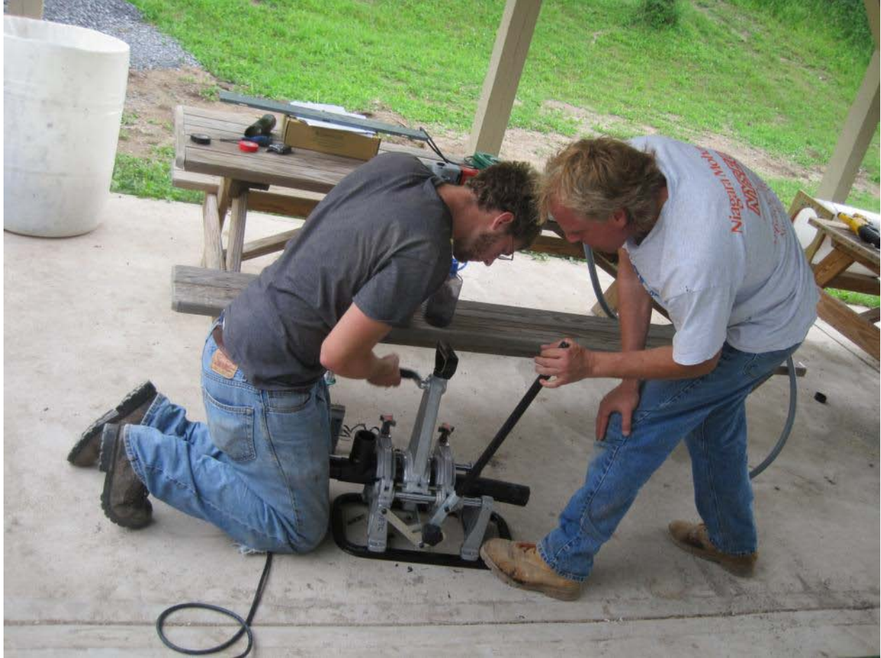
Trimming high density polyethylene to create our distribution manifold to attach to our incoming penstock. Heat fusion is our next step!
