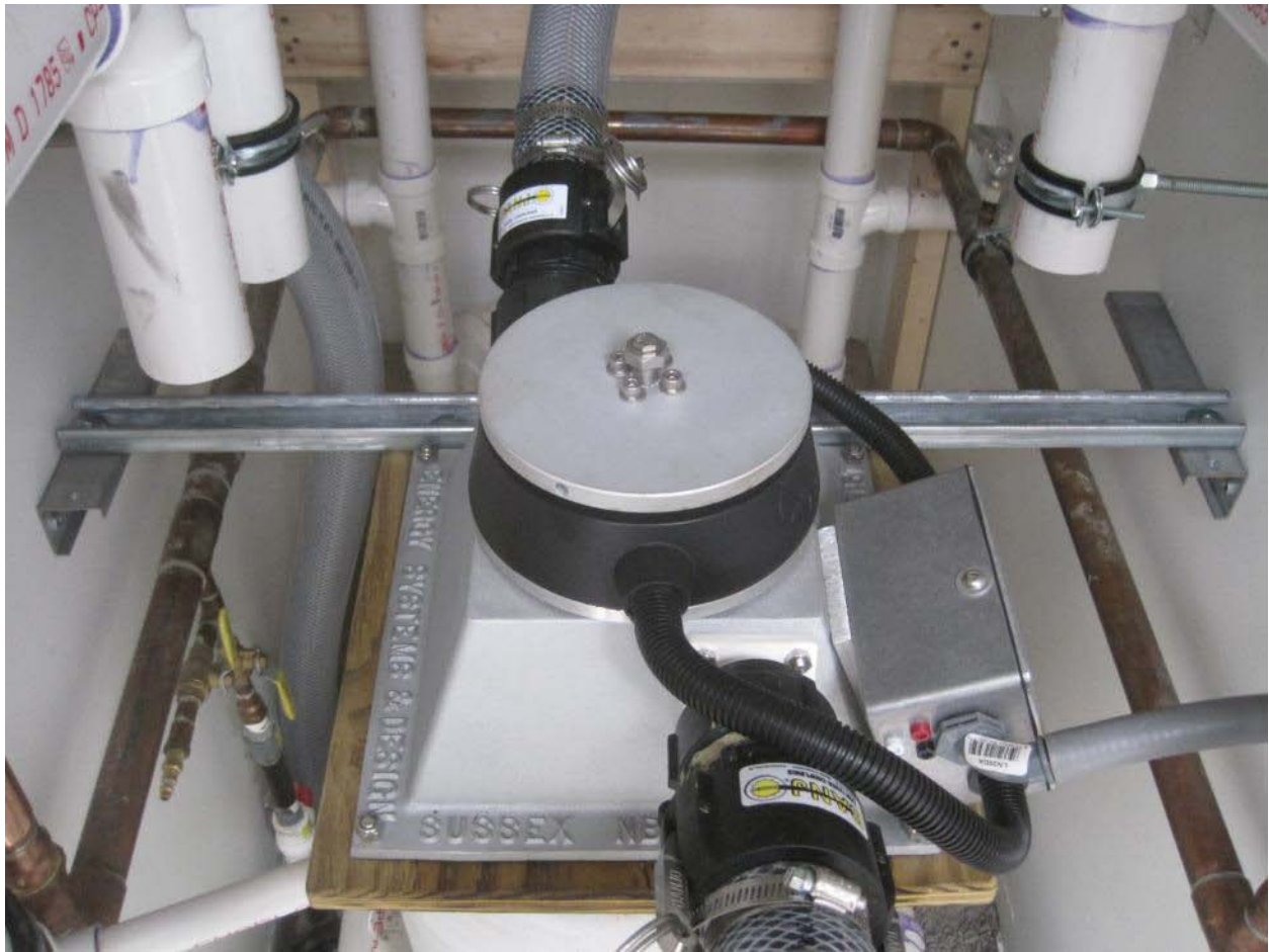
The turbine in its final resting place and ready for action!
