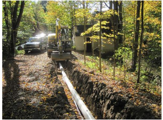
Installing the 8" PVC penstock
