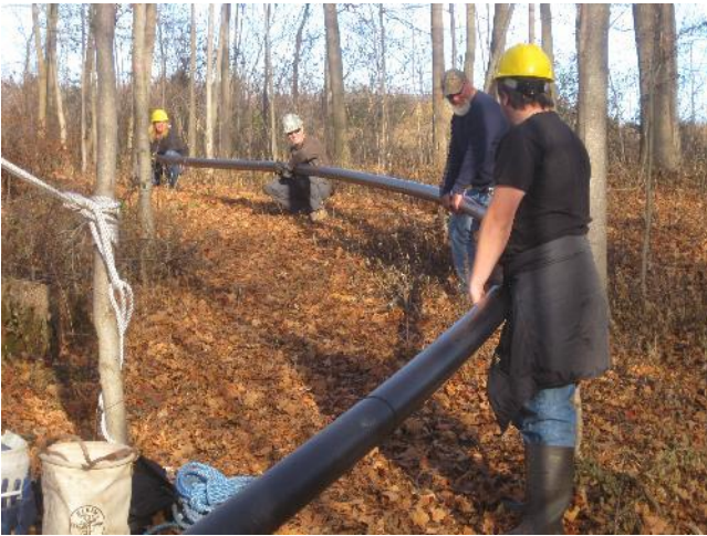
Making a gentle bend with the flexible penstock
