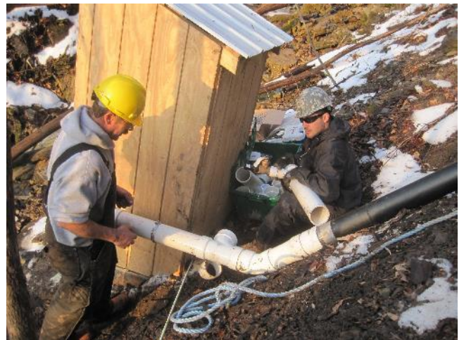
Building the distribution manifold
