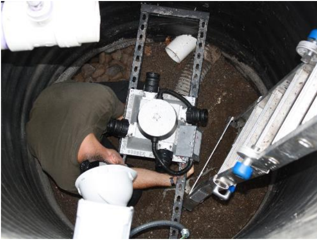
Installing the ES&D Stream Engine turbine
