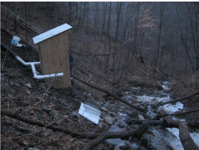
Completed manifold and power house
