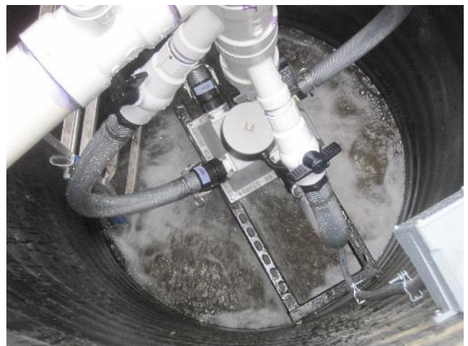
System operating at 350 GPR an 750 Watts (6500 kWh/yr)
