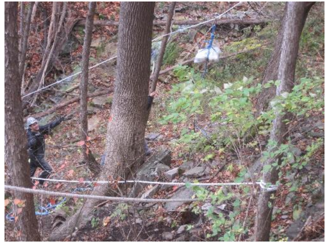
High line transport of concrete on a steep site
