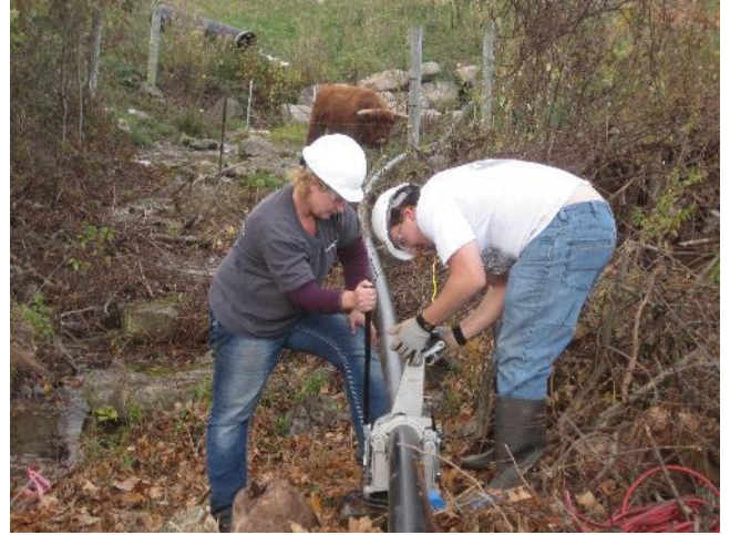
Heat fusion of 4" HDPE penstock
