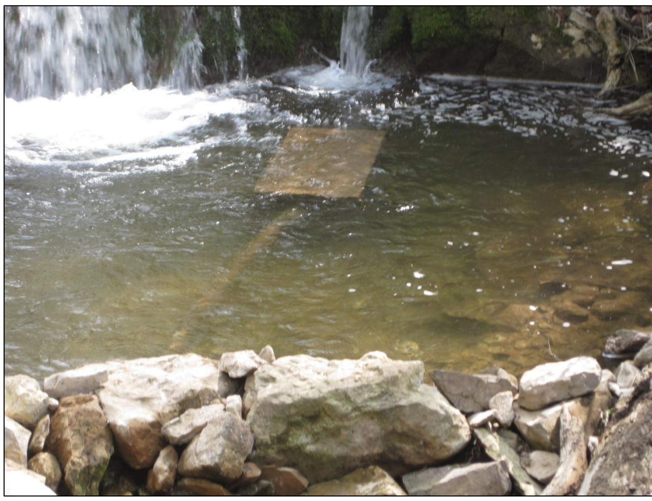
The intake for our system allows only 40 gallons per minute into the penstock pipe
