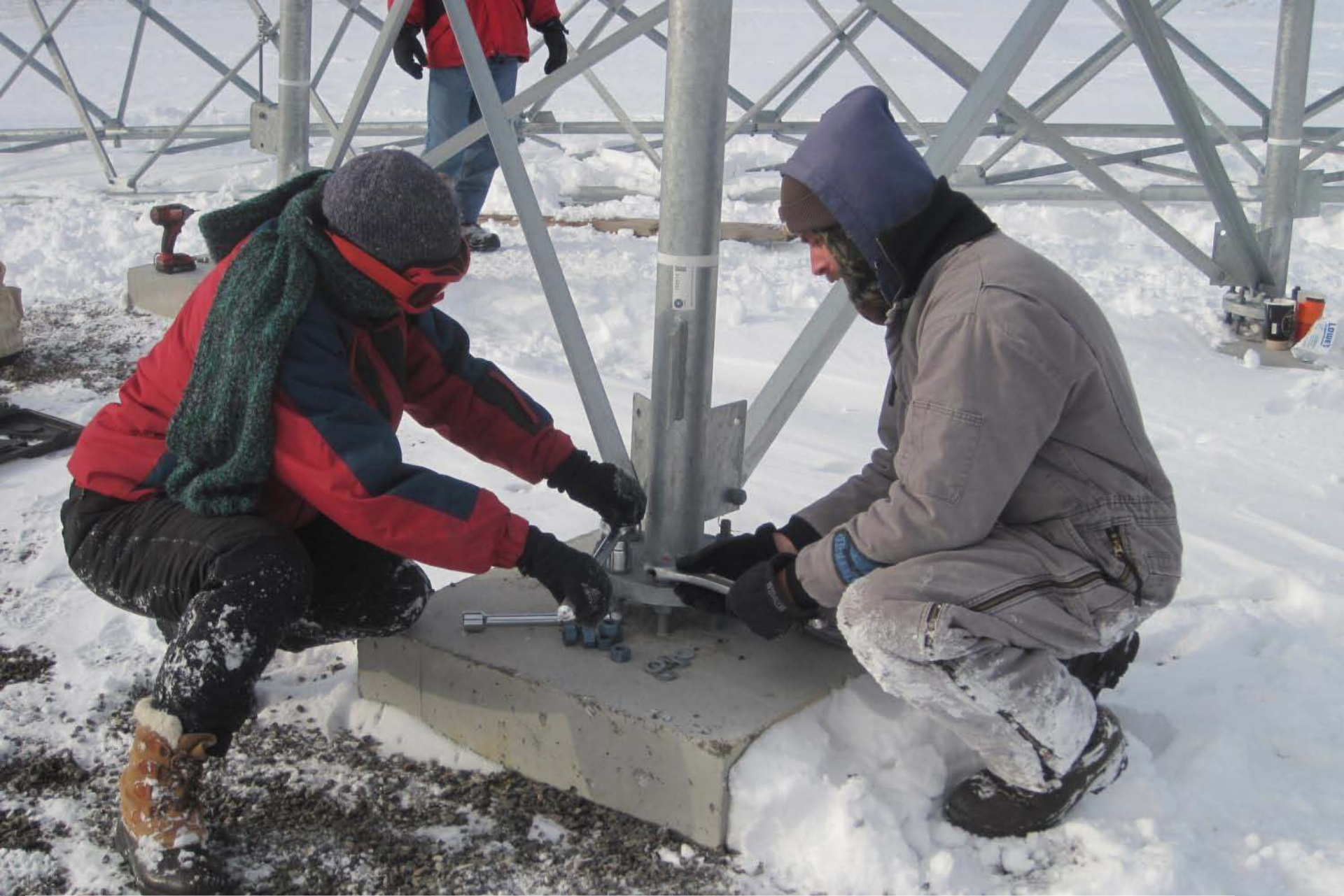
Tightening foundation bolts
