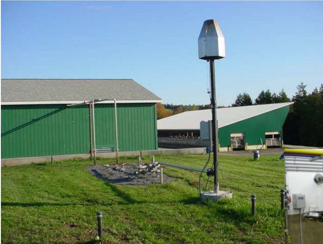
250k gal. plug-flow digester
